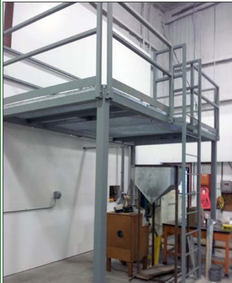
New brush machine and loading platform installed in the Seed House. The platform will accommodate hoppers that funnel uncleaned seed into the machinery
