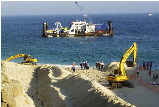
Fig. 4. Installation works of the 2000 FLAG Atlantic 1 in the intertidal area, Brittany, France (courtesy: www.ldravocean.fr).
