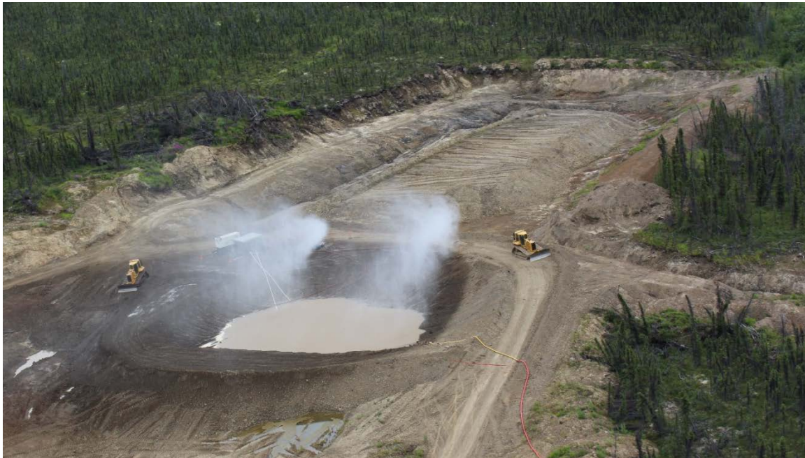
Figure 3-5: Typical Tailings Facility Air Blast Evaporators
