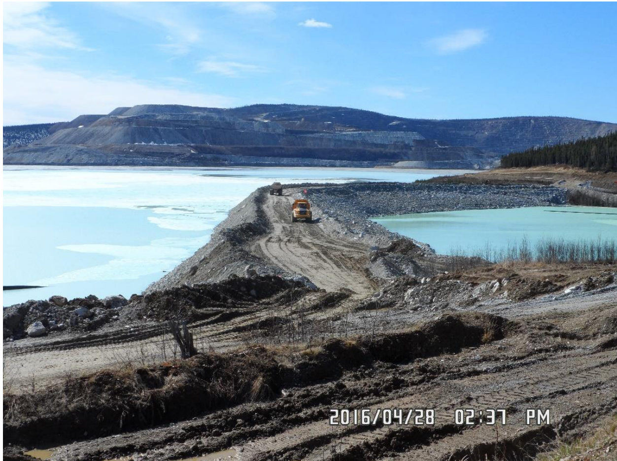
Figure 2-8 - Barge Pond Jetty
