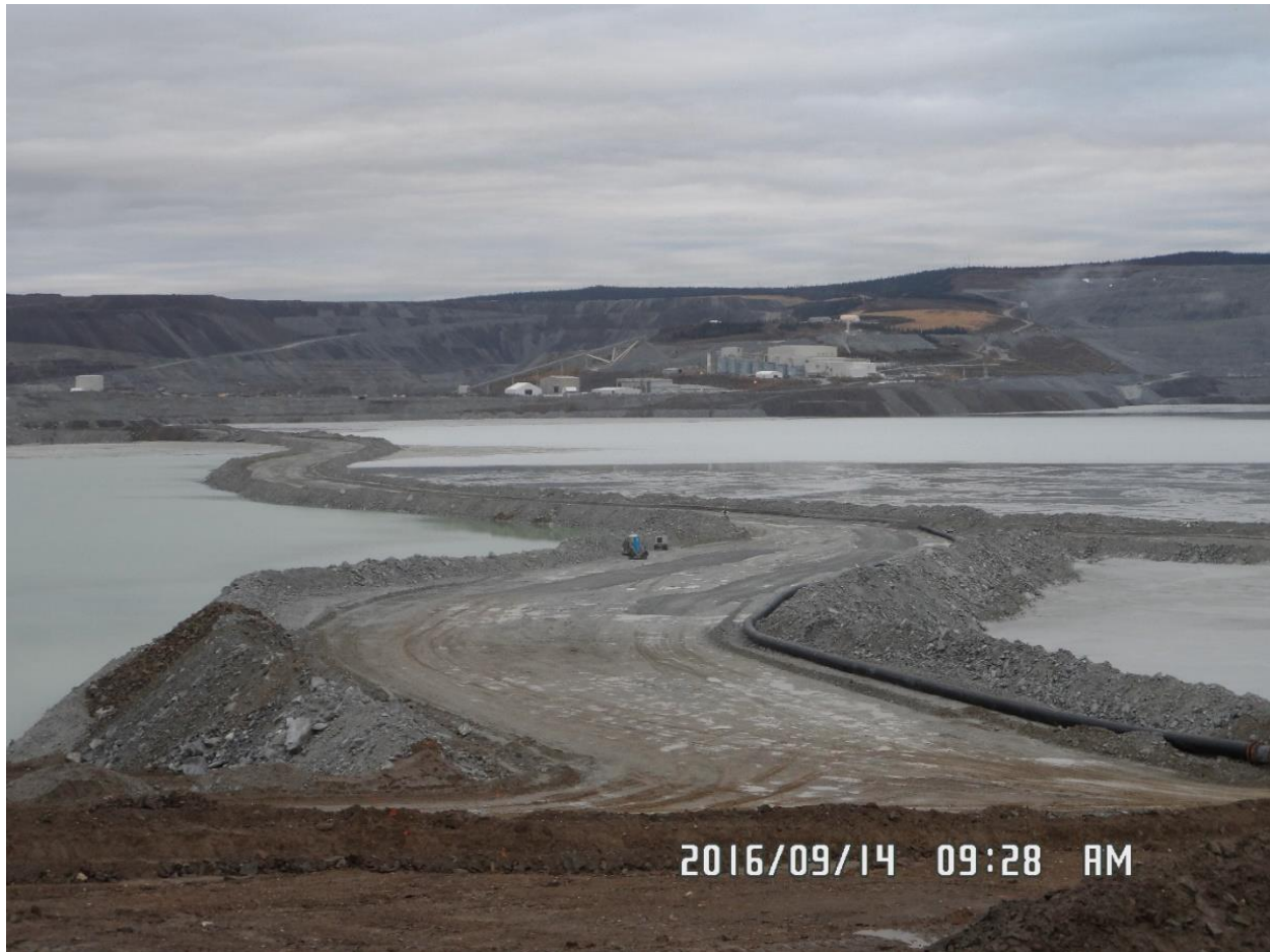
Figure 2-9 - Pearl Creek Causeway Realignment 2016
