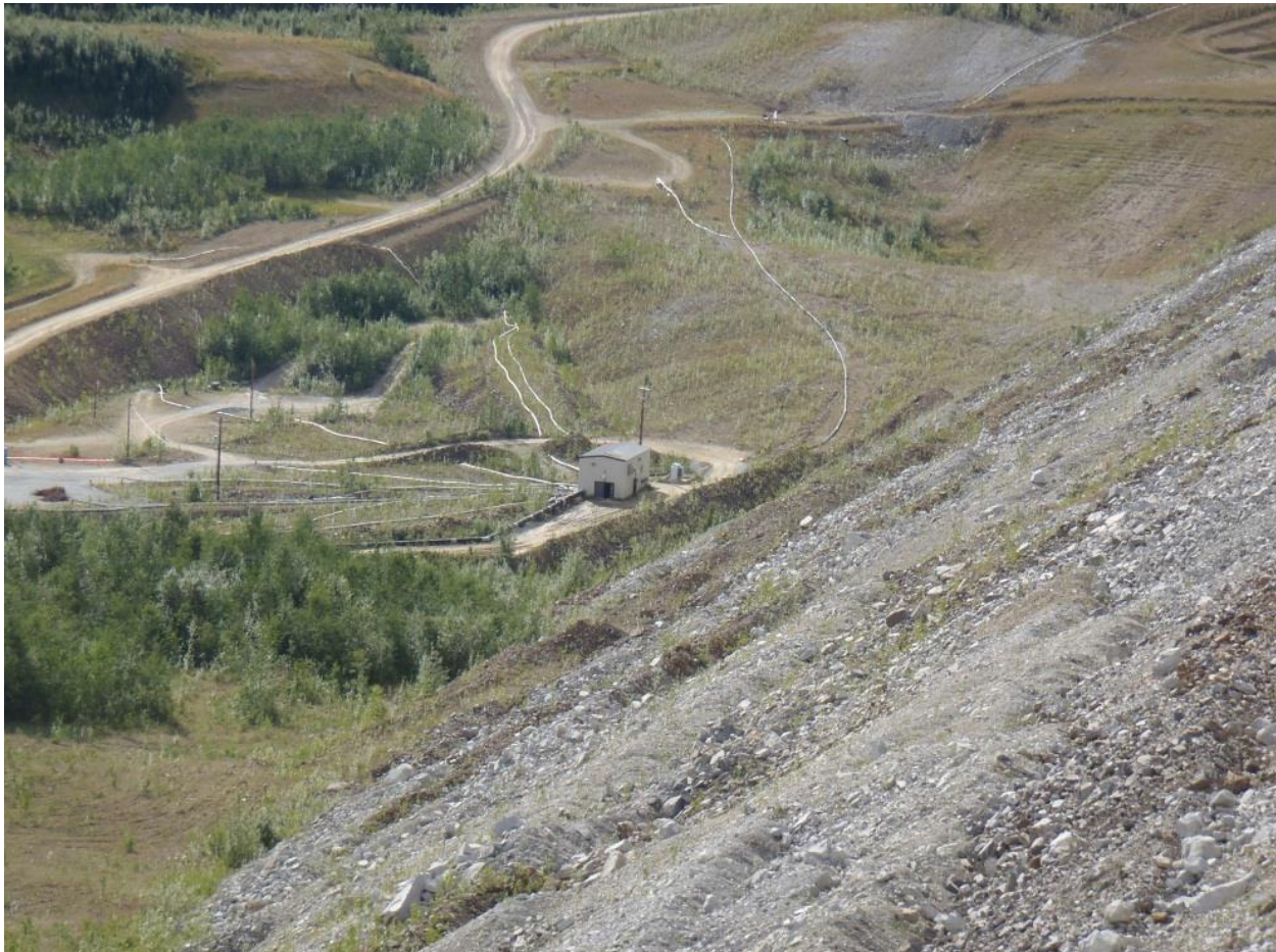
Figure 2-6 - Seepage Reclaim Building
