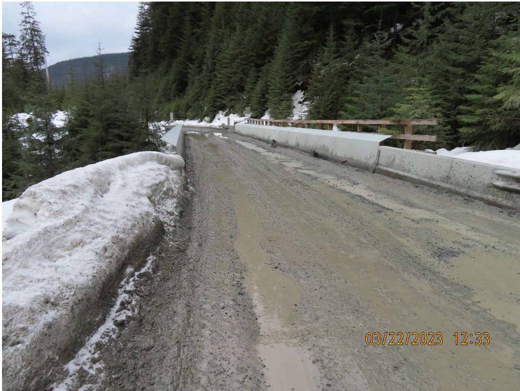
Photo 7. Killer Creek Bridge.
