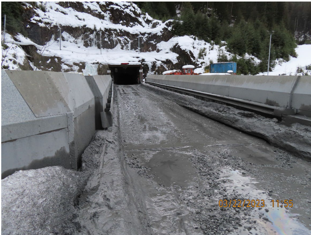
Photo 3. Greens Creek bridge and 920 portal.
