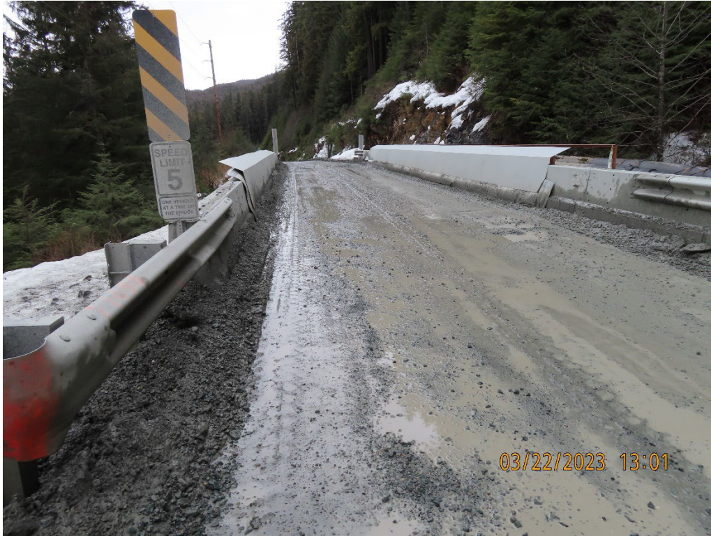
Photo 8. Falls Creek Bridge surface.
