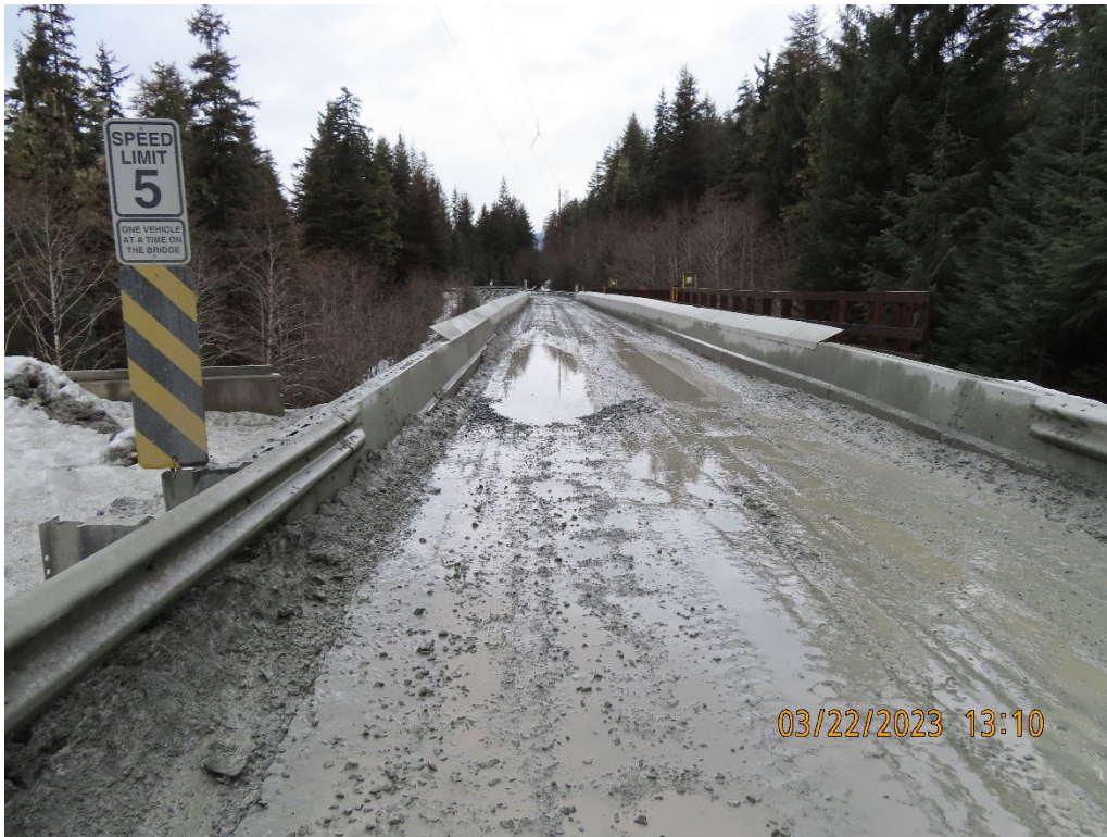
Photo 9. Zinc Creek Bridge.
