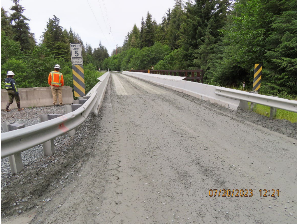
Photo 12. The 3.0-mile marker B Road Bridge (Zinc Creek Bridge).
