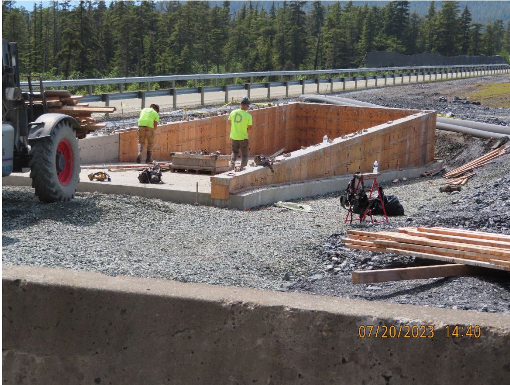
Photo 16. The construction of the TDF degrit basin.
