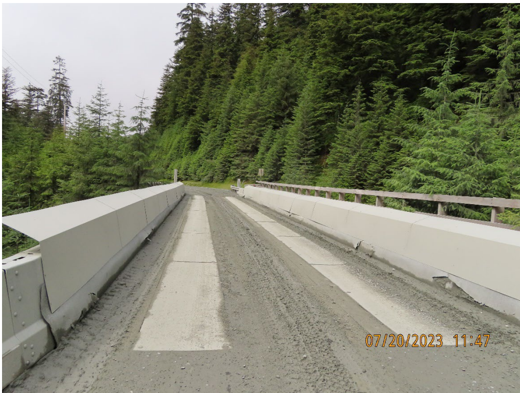
Photo 9. The 7.4-mile marker B Road Bridge (Killer Creek Bridge).
