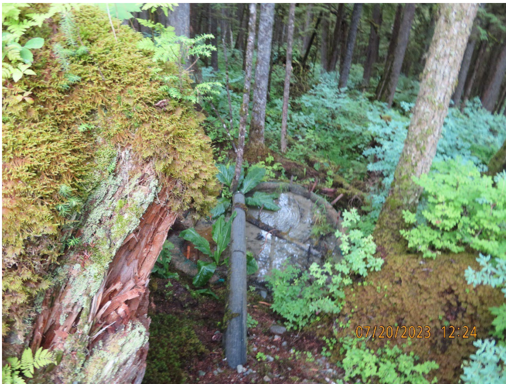
Photo 13. The Gnome Pond outlet pipe.
