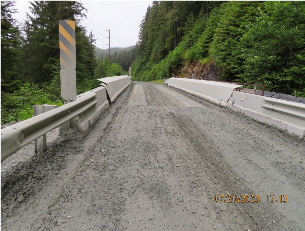
Photo 11. The 3.4-mile marker B Road Bridge (Falls Creek Bridge).
