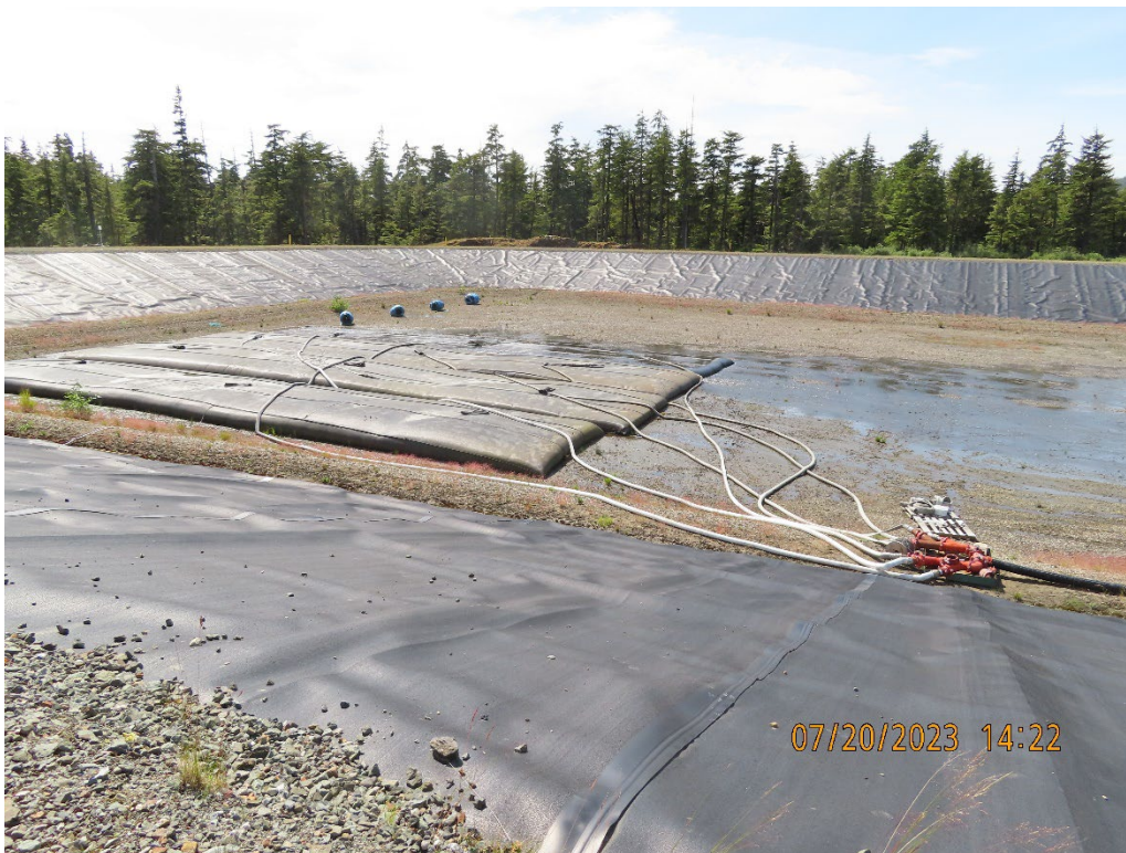
Photo 15. Pond 10 with dewatering bags temporarily staged inside.
