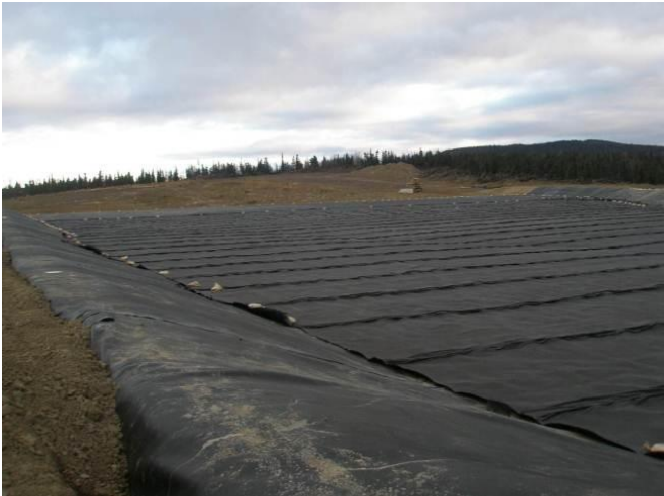
Figure 20: Liner Placement on the FTDS
