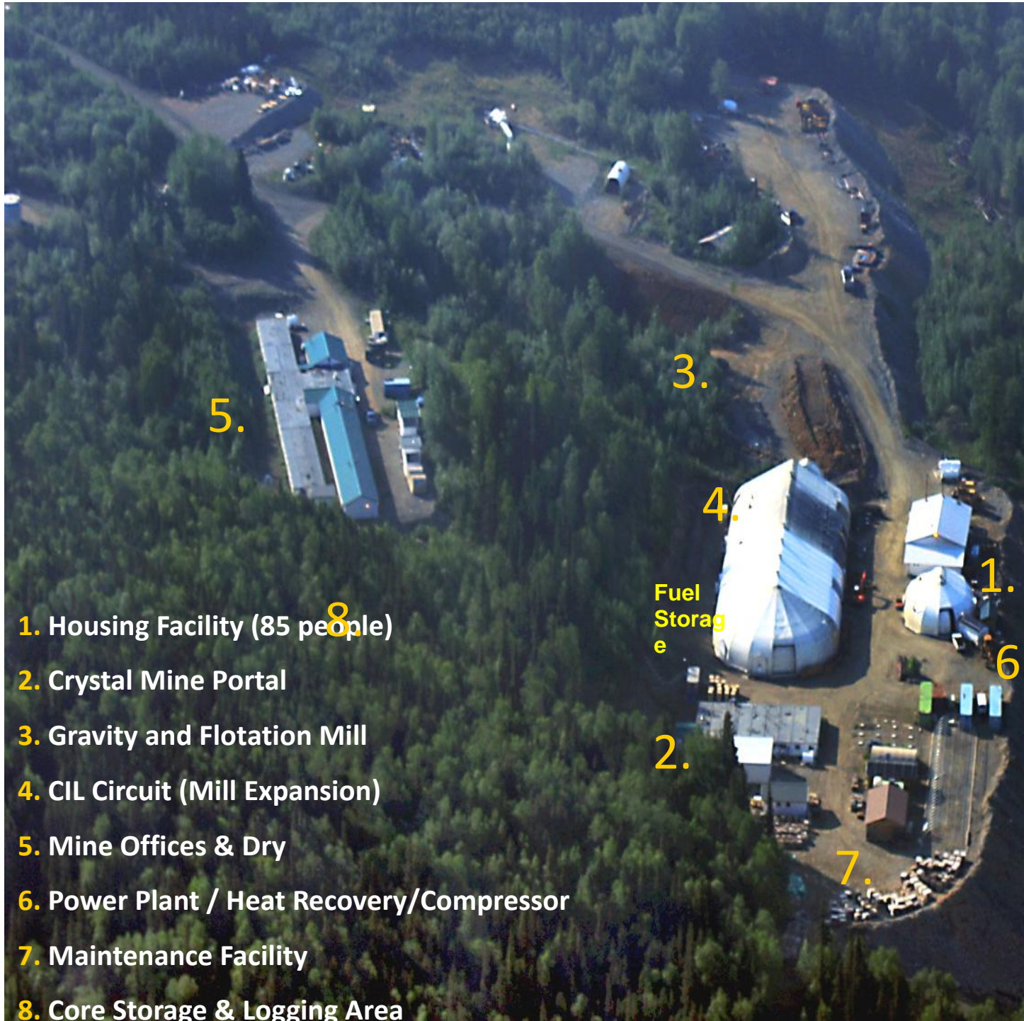
Figure 6: Aerial Photo of the Nixon Fork Mine (Looking South)
