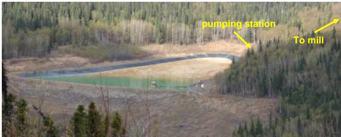
Figure 17: Tailings Storage Facility (Looking North)
