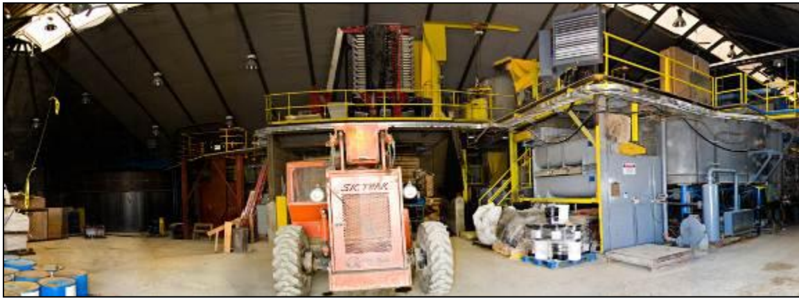
Figure 7: Gravity and Flotation Mill (right) and CIL Circuit Area (Left)
