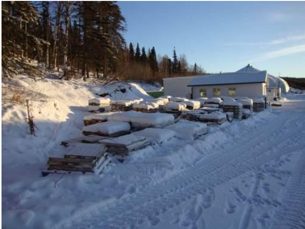
Figure 14: Process Water Recycle Tank Location (Looking Southeast)
