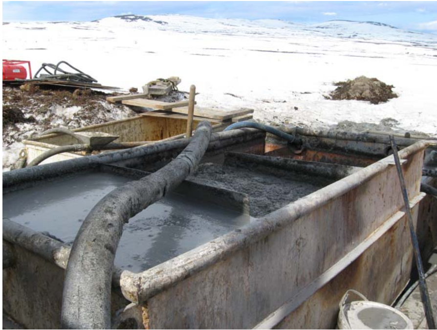
Figure 3. Drill rig number 2, settling box for recycling drilling muds.
