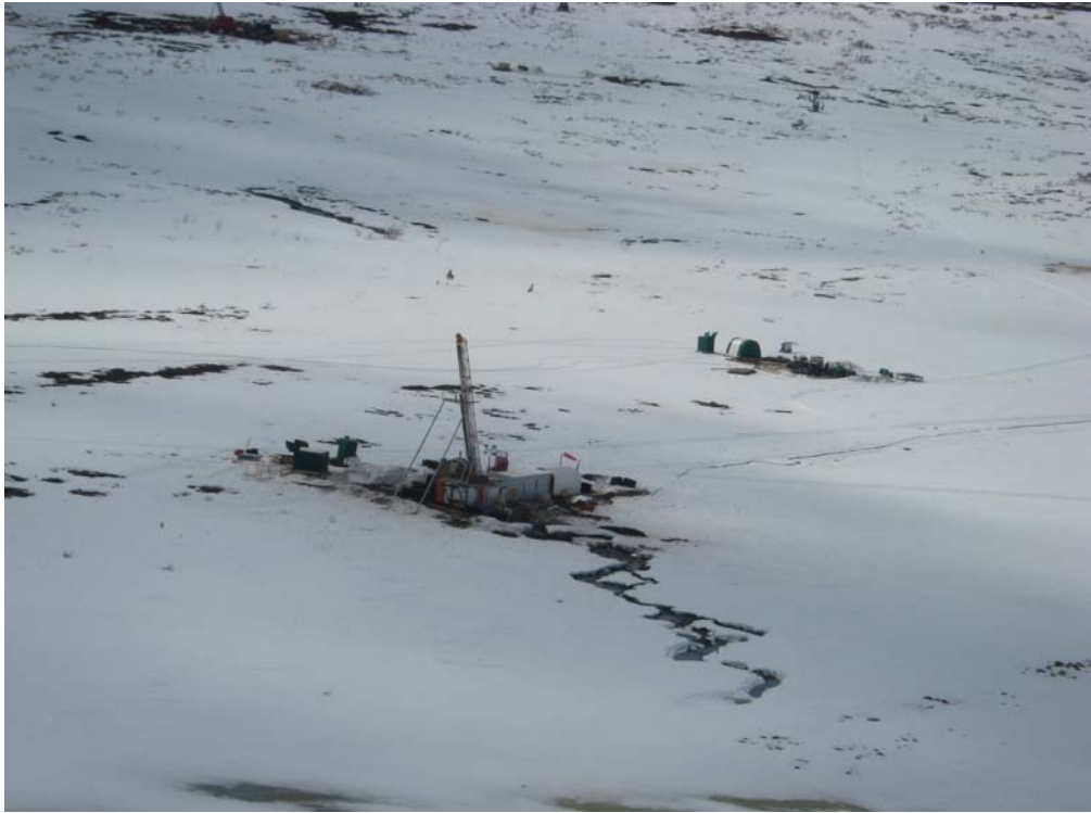
Figure 2. Drill rig number 2.
