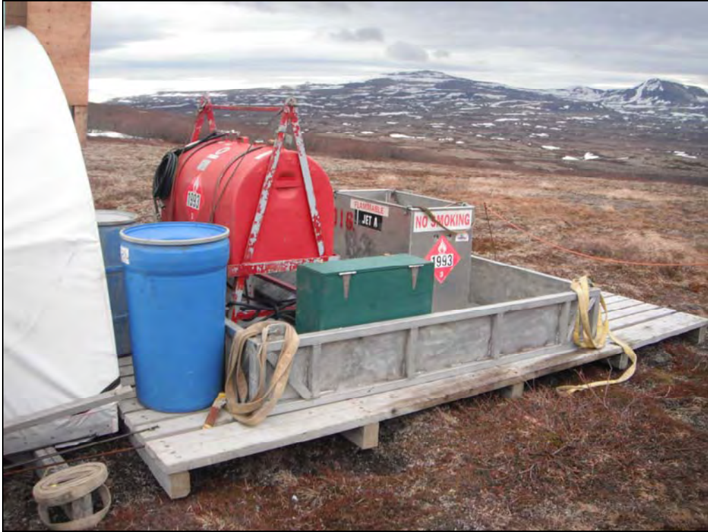
Figure 5. Fuel storage in catch basin on tundra pad, with spill kit and scrubbers (blue bin).
