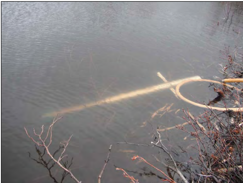
Figure 8. Screened water intake submerged in beaver pond.
