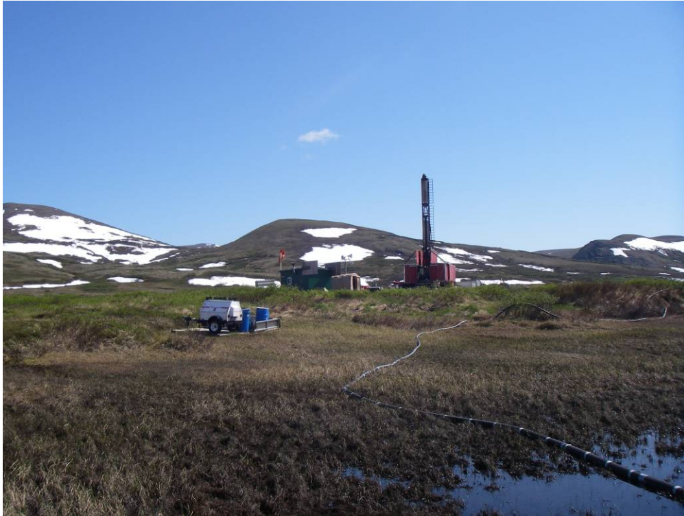
Figure 3. Drill rig 8407 (No. 5).
