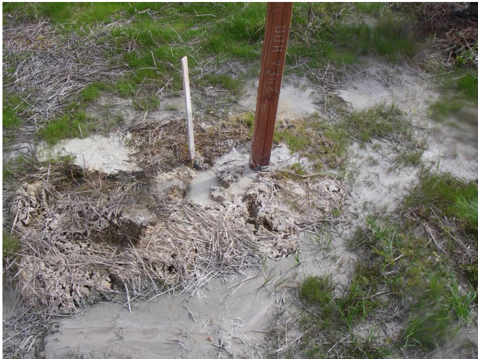
Figure 16. Water discharge from drill hole, reclamation site 7362.
