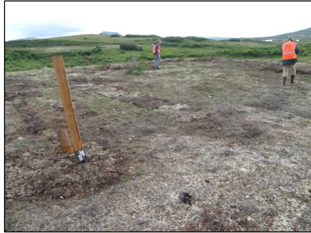
DDH12555 site reclamation in progress.
