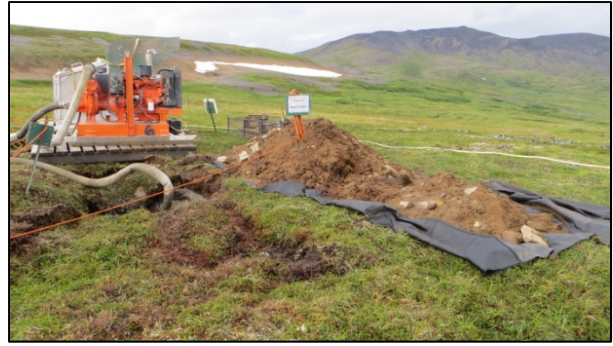
Sump and material stockpile for GH 13374
