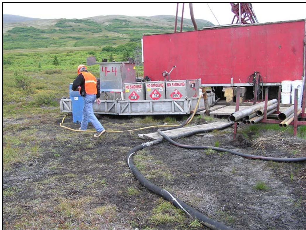
Figure 12: There was a slight fuel odor near the fuel tanks for Drill Rig # 2 and a little staining on the ground.
