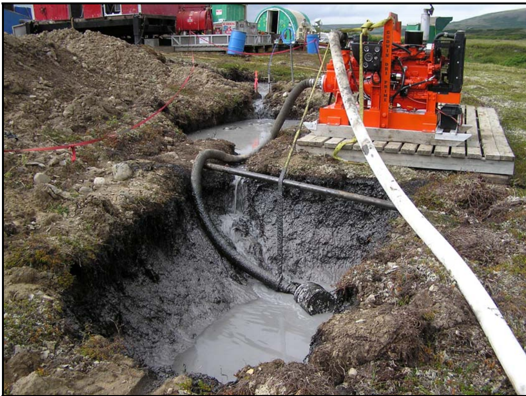
Figure 16: Drill Rig # 5 sumps.
