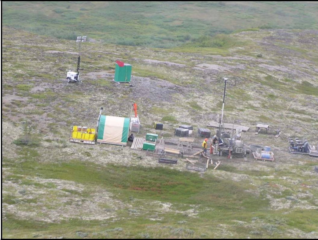
Figure 1: Drill Rig # 8 - Geotechnical drilling rig at hole number P-08-87.
