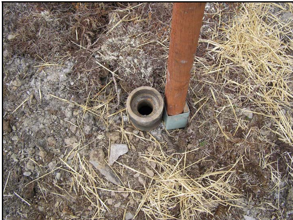
Figure 33: DDH No. 8415 - unable to determine if hole was plugged.
