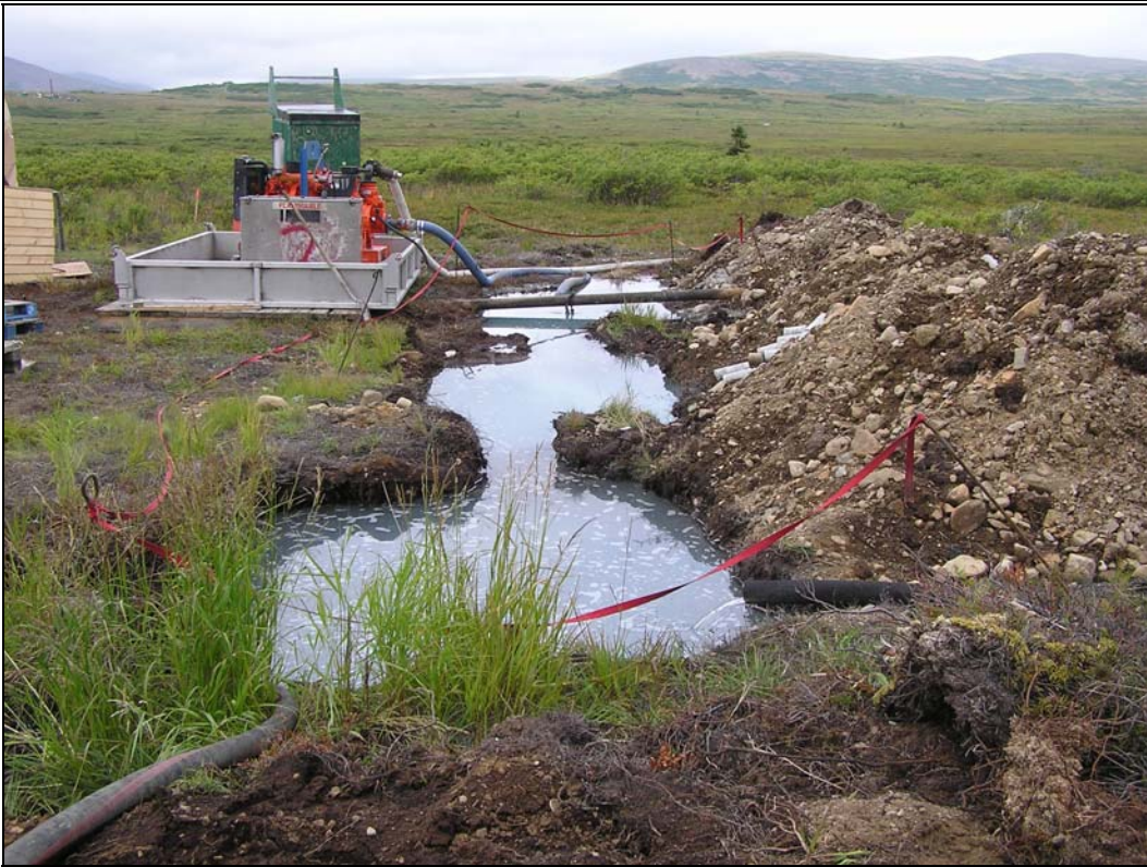
Figure 13: Sumps at Drill Rig # 2.
