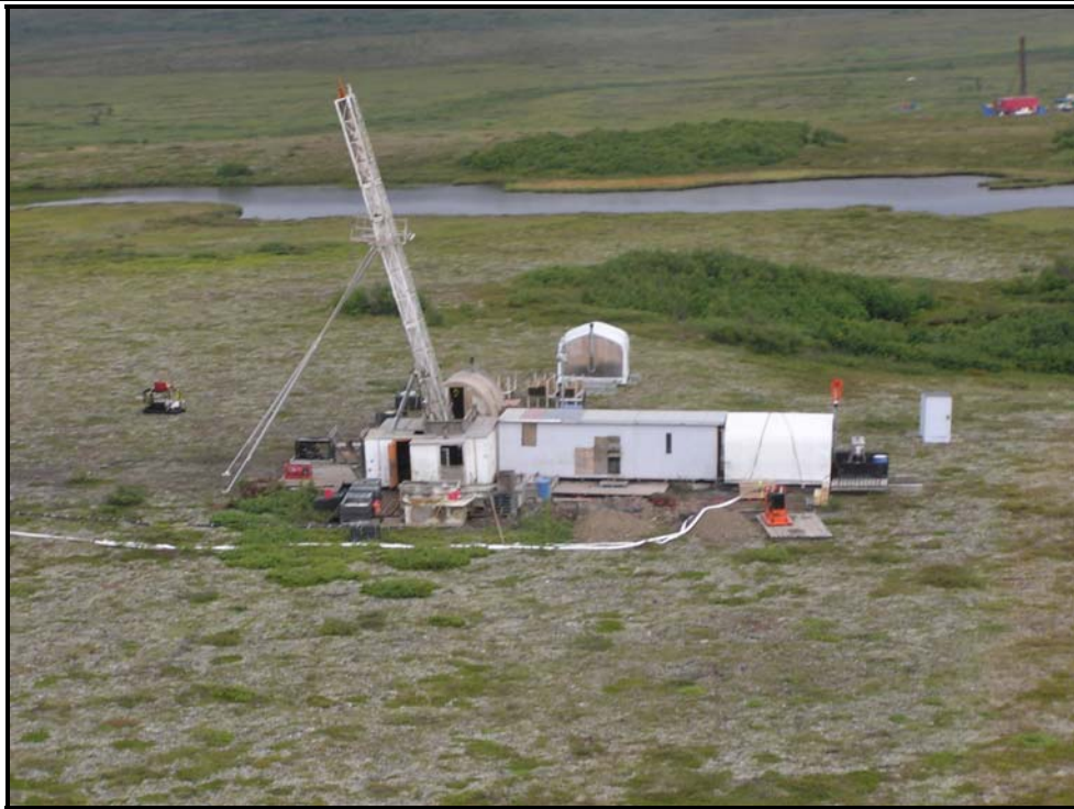
Figure 21: Drill Rig # 1 on drill hole No. 8422.
