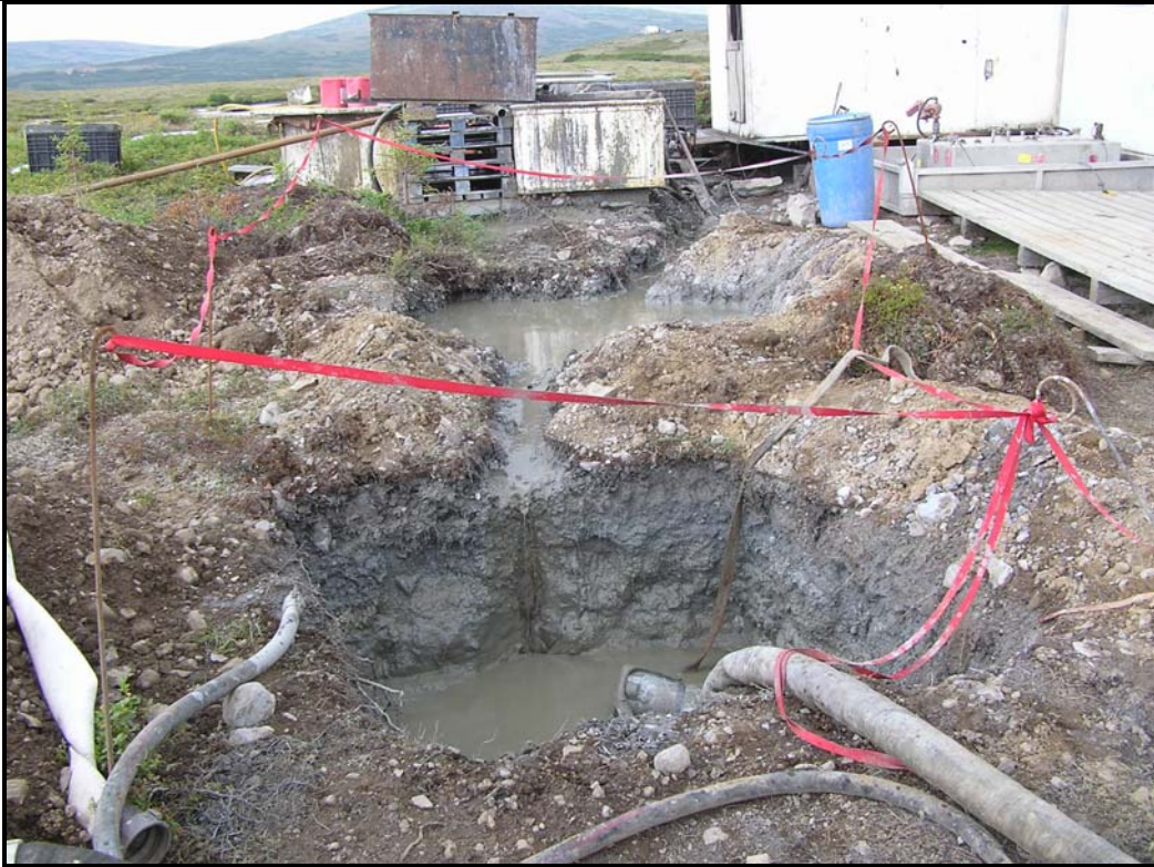
Figure 23: Sumps at Drill Rig # 1.
