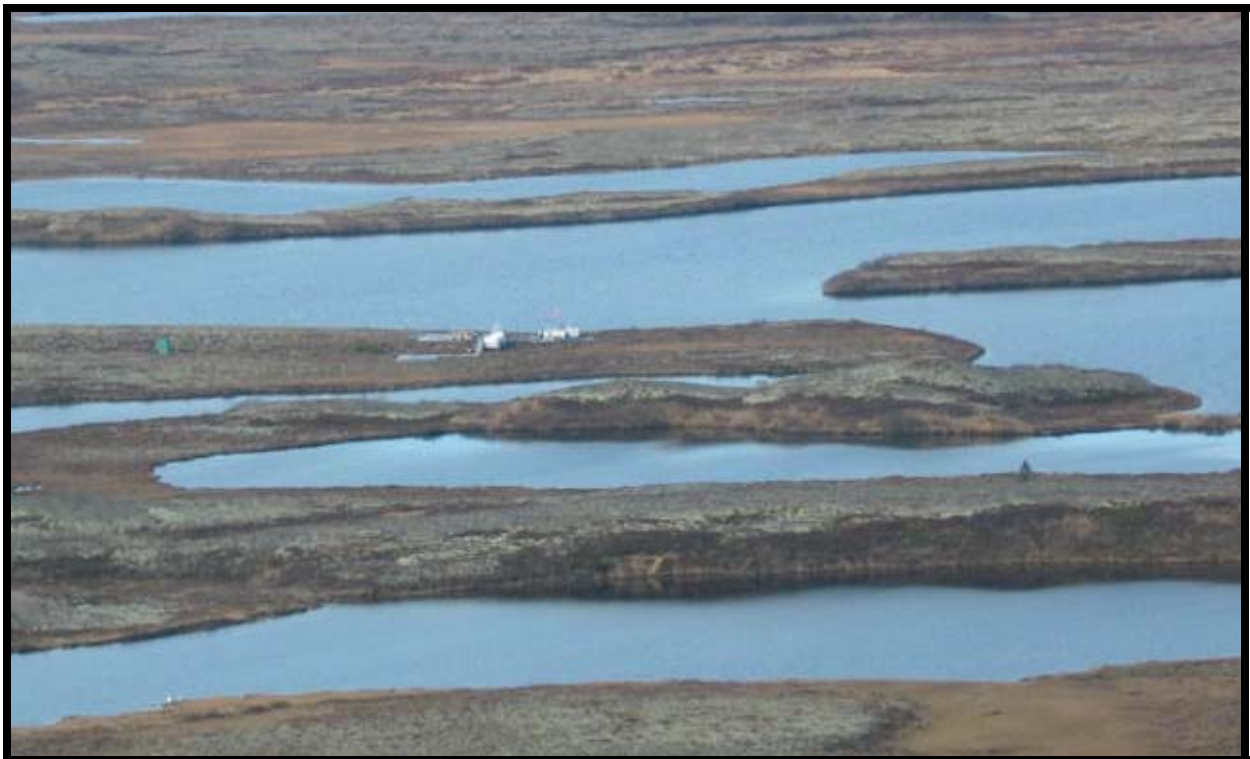
Figure 16: Big Wiggly Lake and Fuel Storage Facility
