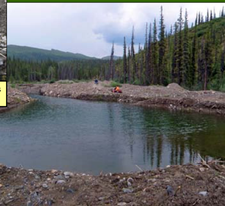
Stabilized tailings pond on California Creek allow for natural re-vegetation.
