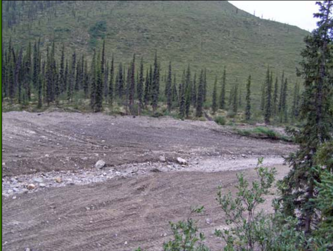
Re-contoured embankments blends with surrounding topography
