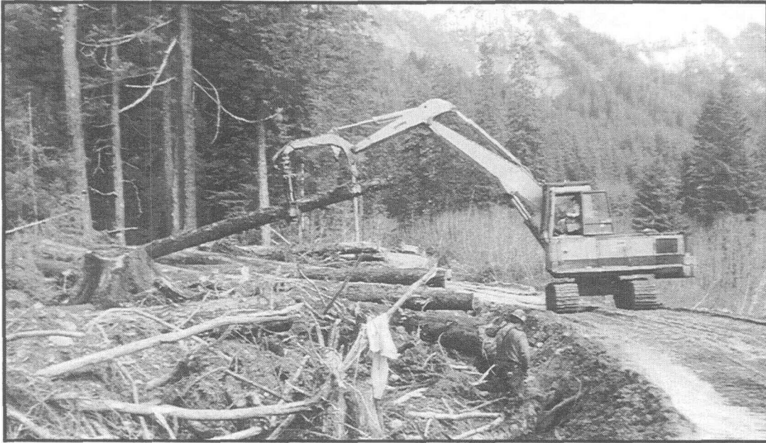
Log picker on road west of Icy Cape log transfer facility
