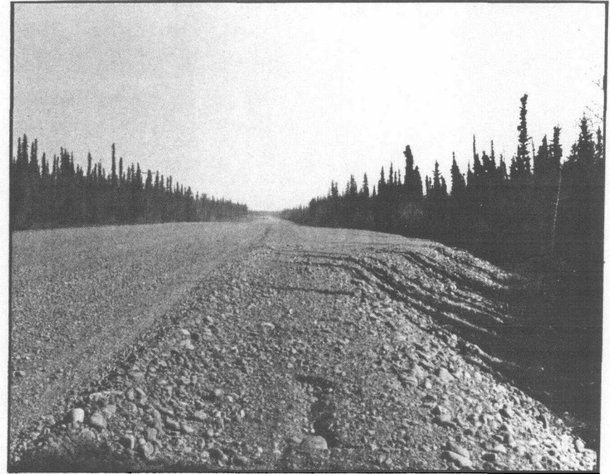
The wide, straight highway alignment creates a relatively monotonous view of this landscape.
