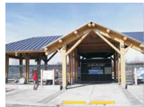
Figure 9. South Palmer Station Structure
