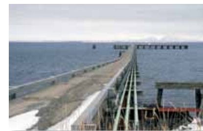
Cold Bay city dock
